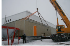
•Wood pellet boiler being unloaded at YK City Pool & Arena.
